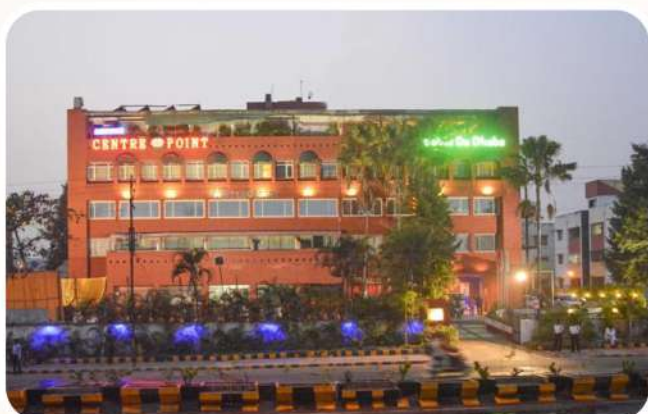
Hotel Airport Center Point, Nagpur
